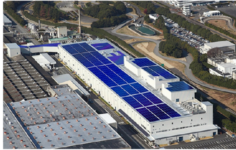
Mitsubishi built this rooftop solar plus storage system.
